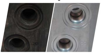
Plate Heat Exchanger cleaned
